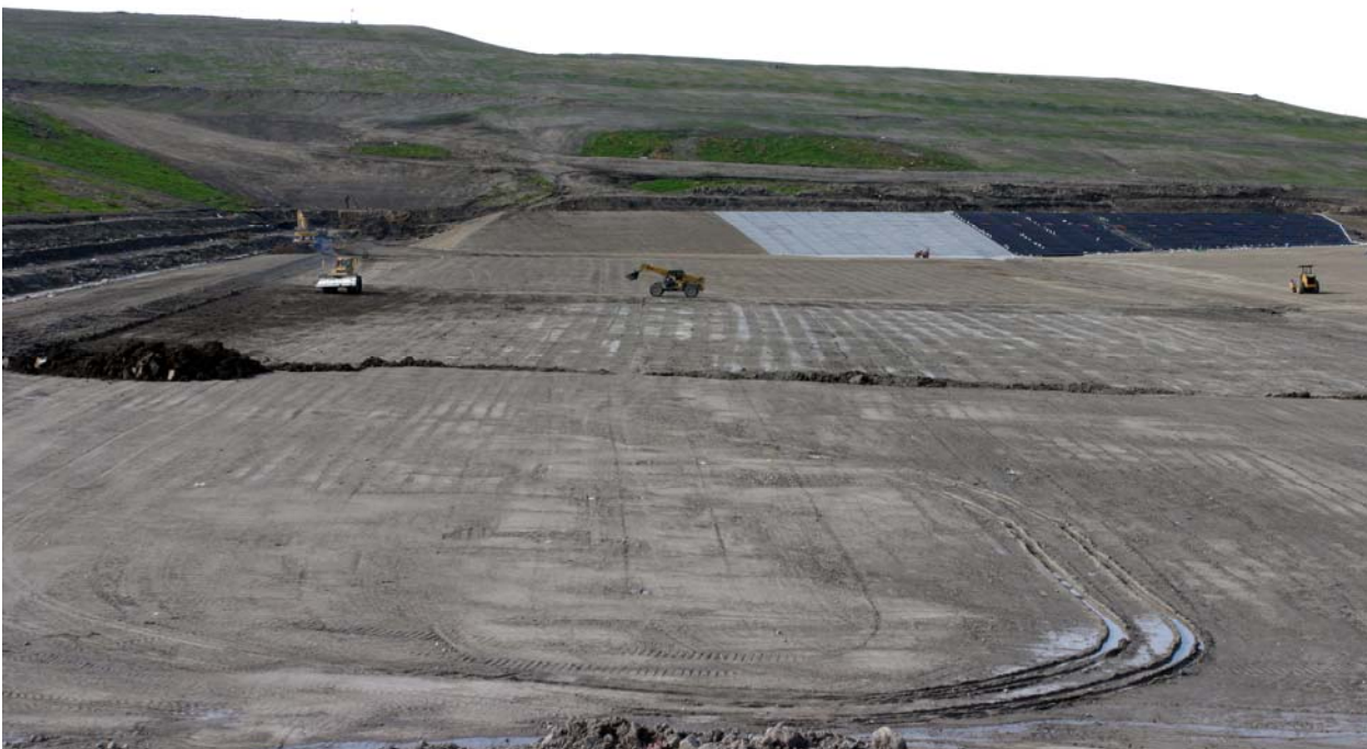
Carleton Farms Landfill, Cell 237 Sub-Base Construction, Sumpter Township, 2007.
