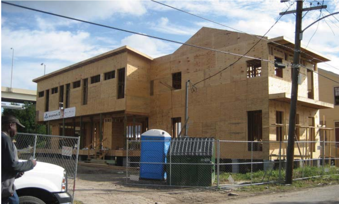
Figure 5: Construction 2 (Source: Authors).
