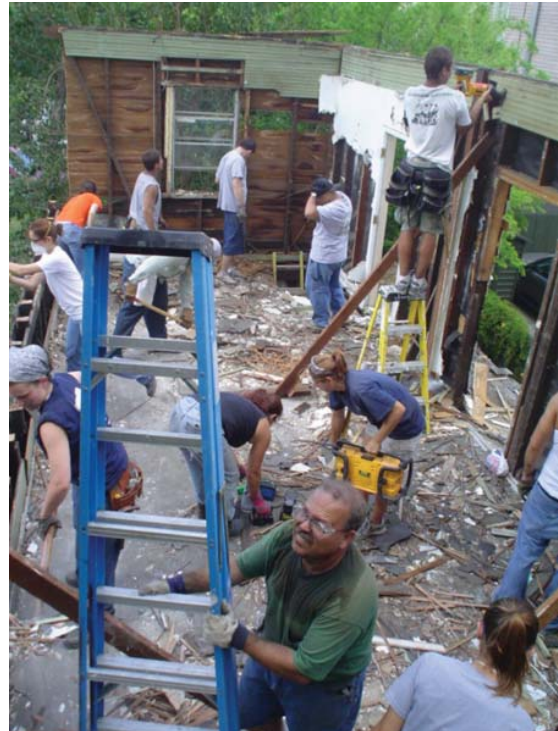
Figure 2: Site Demolition and Assessment of Building Materials for Re-Use (Source: Authors).
