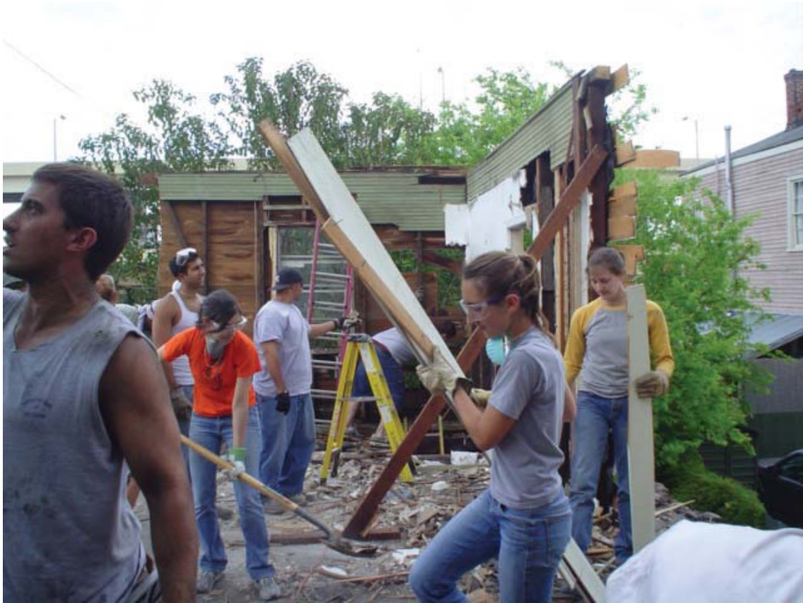
Figure 3: Site Demolition and Materials Re-Use Assessment (Source: Authors).
