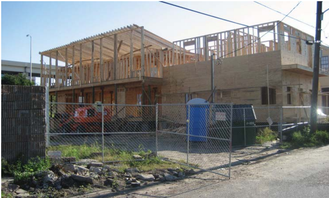
Figure 4: Construction 1 (Source: Authors).
