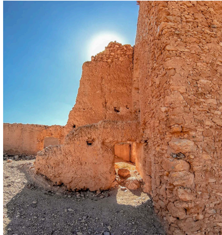
Abandoned rammed earth village outside of Marrakech
