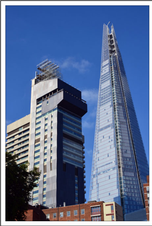
Figure 7. The St. Guy's Tower Retrofit Project (2014), London, UK, by Penoyre Prasad Architects and Arup features new exterior cladding and restoration of a landmark 1970s NHS hospital. Photograph by George Rex.
