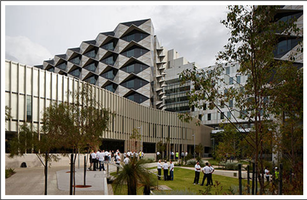
Figure 2. Fiona Stanley Hospital, Brisbane Australia (2014) by Hassell with Silver Thomas Hanley, is a large state government hospital and teaching facility with a four-story rehabilitation hospital. The rehabilitation hospital has an integrated therapeutic landscape where exercise and outdoor activities are central to the recovery process. Designed landscape elements such as kerbs, slopes, varied surfaces, and paving textures helping patients practice and challenge themselves outdoors to aid in their recovery. Photograph by Peter Bennetts.
