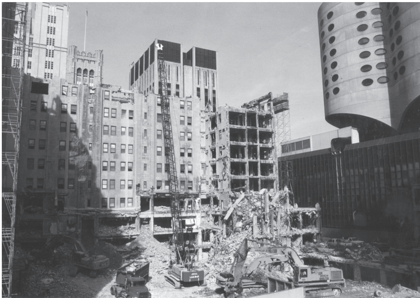
Figure 3. Passavant Hospital demolition, Chicago, 2001.
